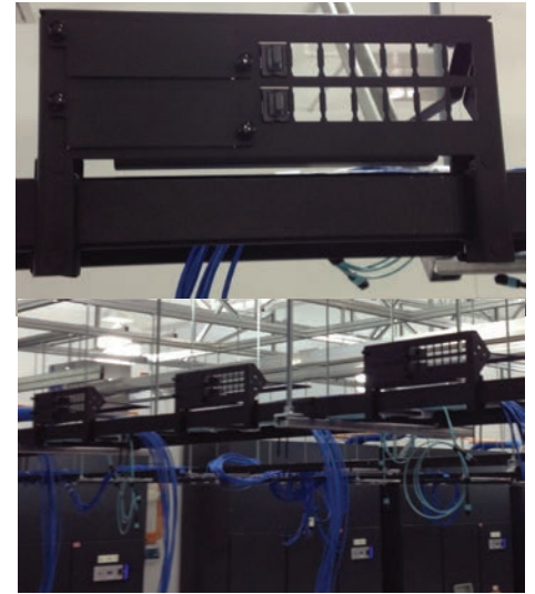
Overhead Pathway Racks. 架空衔接机架
